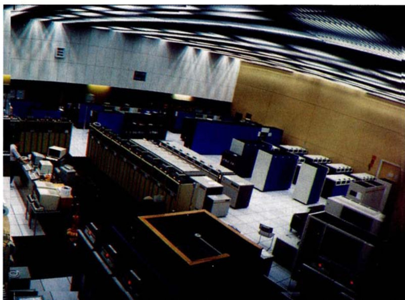
era of the combined service provided by IBM and Siemens. (Courtesy Chris Jones.)
